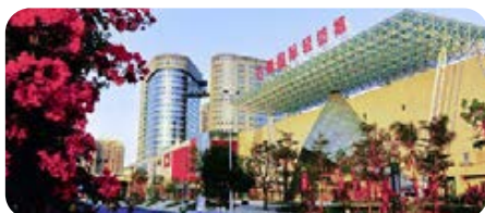
Nanhu Road, Shishi City, Fujian Province
